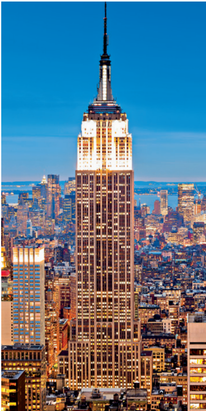
Otis is refurbishing and modernizing the elevators in the Empire State Building, still one of the world's most famous office buildings more than 80 years after Otis installed the original equipment.
